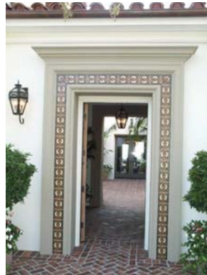
Entry Surround Detail
