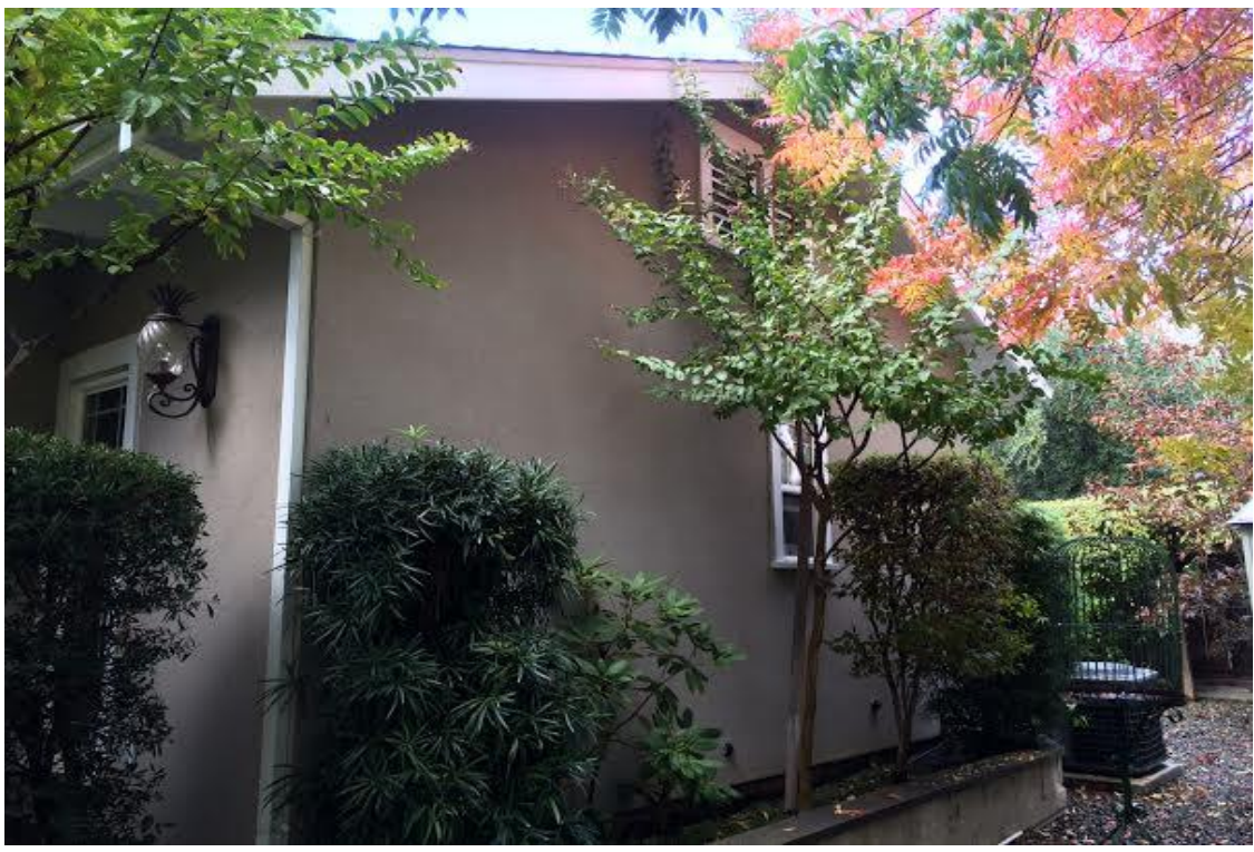
3. Pool House Right Side – South Side
