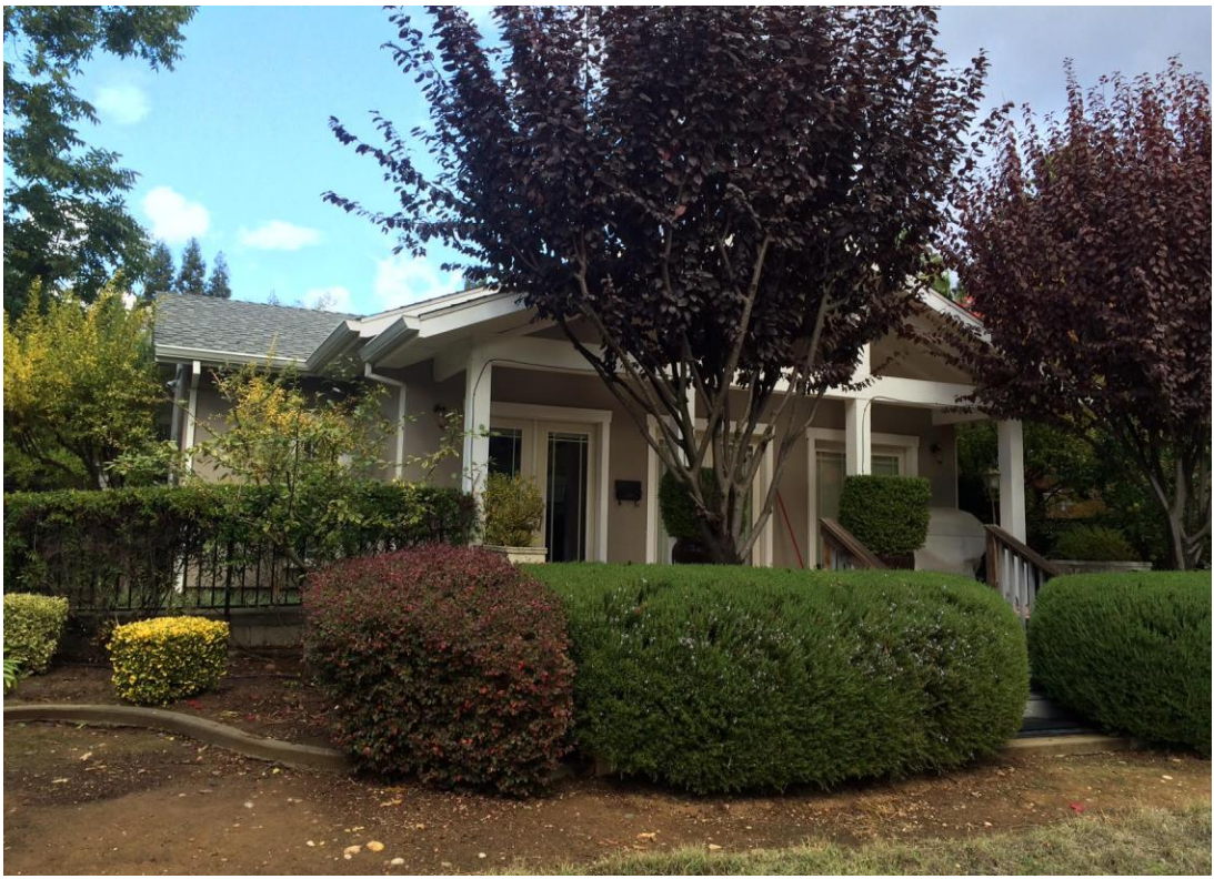
1. Pool House Front – West Side
