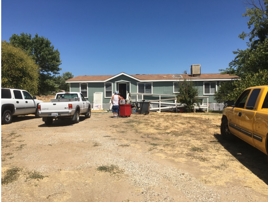
Photo 2: View east of the west elevation of Building 5.
