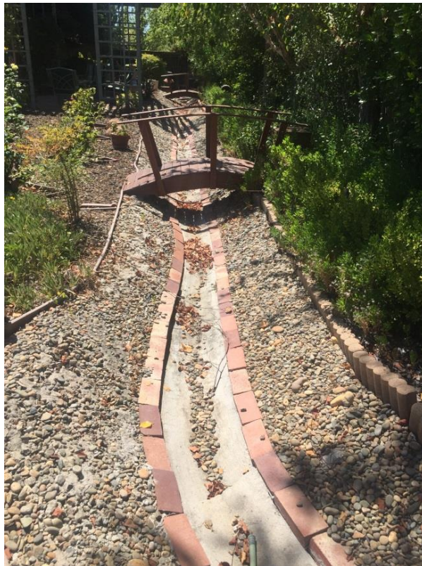
6. View of the drainage ditch located on the neighbor's property (APN:122-0480-012).
